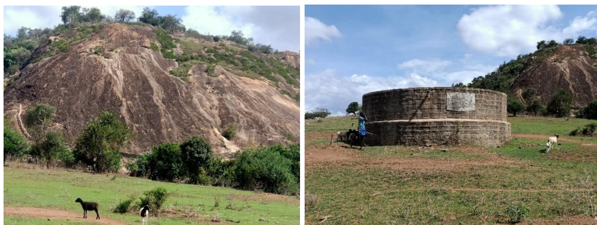
Plate 9-8: A Rock Catchment and Community Storage Tank
